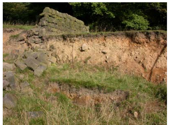
Landslip above Lobb Mill in 2005
