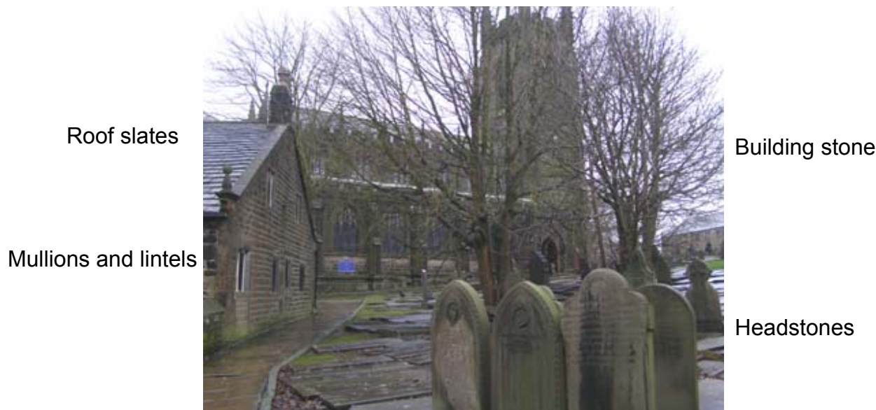
Heptonstall churchyard to show the use of local sandstones
